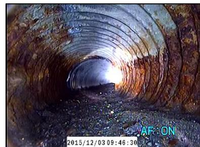
*These corrugated metal pipes (above – Concord Rd culvert and below – drainage pipe) need replacement.*
