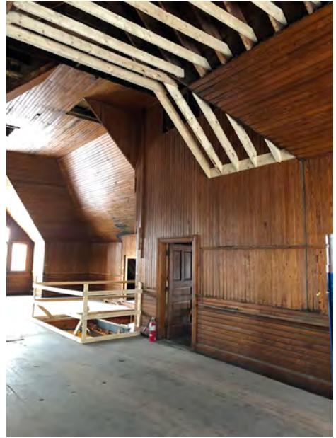
Southwesterly View of Third Floor
