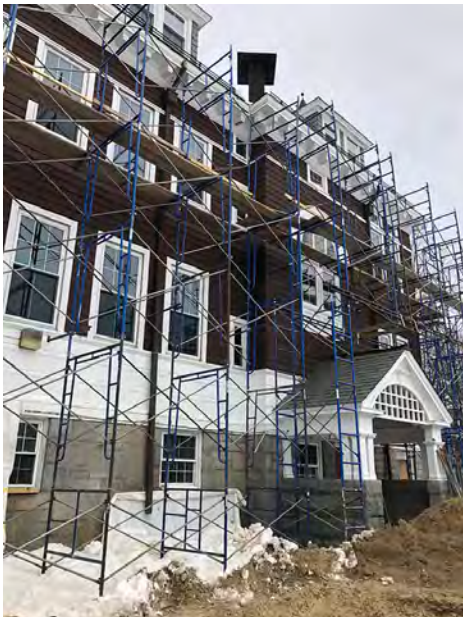
Scaffolding Installation at East Facade
