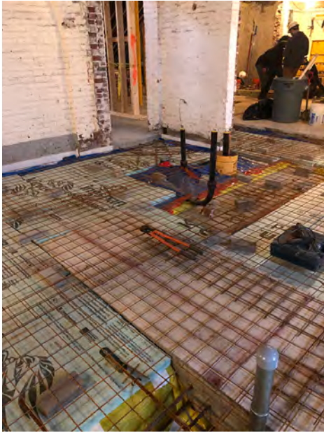
Looking Northwest from Electrical Room and Across Men's Room Area
