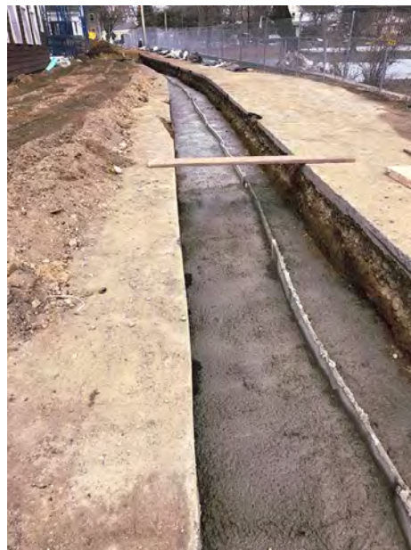
Concrete Coverage over Conduits Completed
