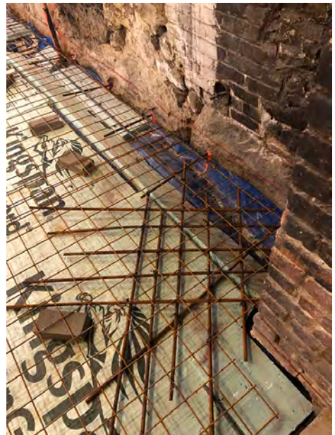
Typical Reinforcement at Corner of Slab
