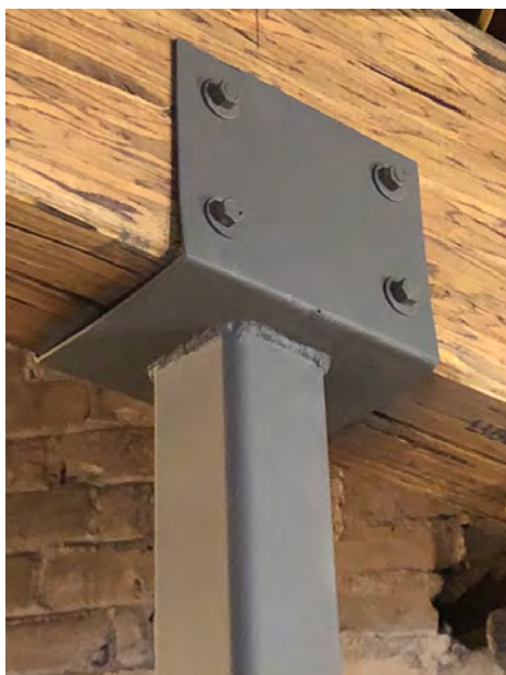
Tube Steel Post and Cap Supporting Added Beam in Basement at Facility Manager's Office
