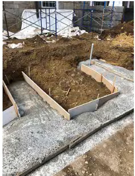
Concrete Coverage in Place at Conduit Feeds into the Building
