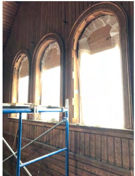
Tripartite Windows at Front Facade of Third Floor Removed Offsite for Repair and Restoration
