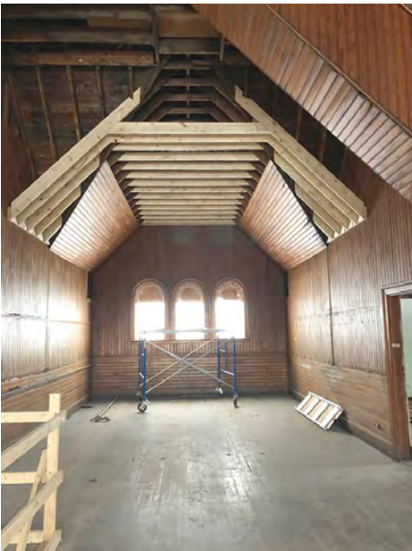
Collar Tie Framing at Height of Former Ductwork Frames Ceiling Shape of Seminar Room
