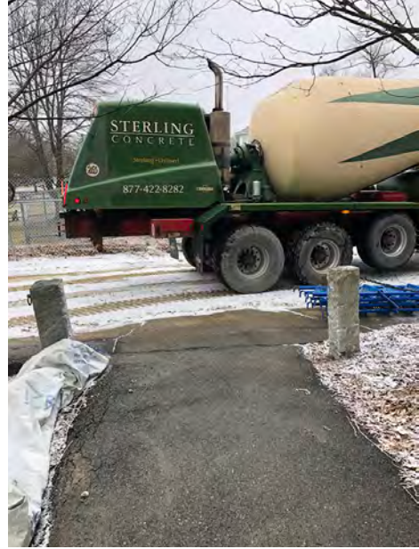
Concrete Delivery for Placement into East Half of Reconfigured Basement Level
