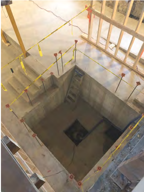
Elevator Pit at Lower Lobby
