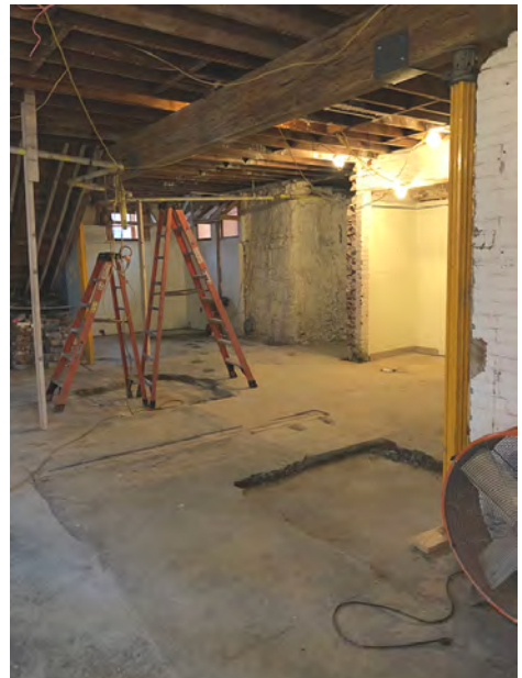
Northwestern Portion of Basement at Community Education Area
