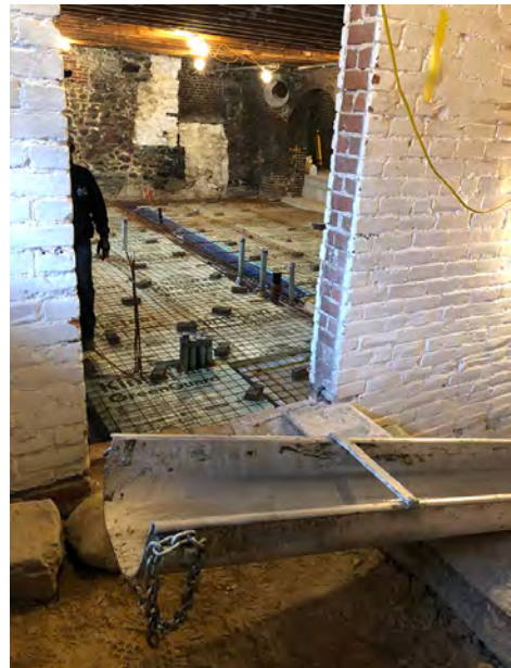
Looking South from East Portico Entrance Toward Electrical Room and Boiler Room Areas
