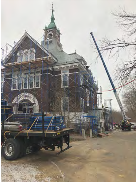
Commencement of Scaffolding Installation at Exterior of the Building
