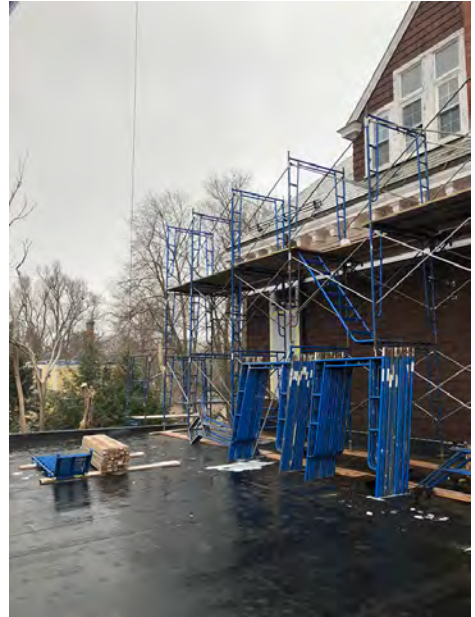
Scaffolding Delivery to Rear Facade at Gym Roof
