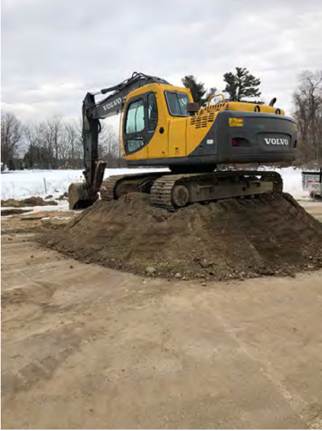
Excavator in Position for Preparation of Grading for Placement of Transformer and Generator Pads
