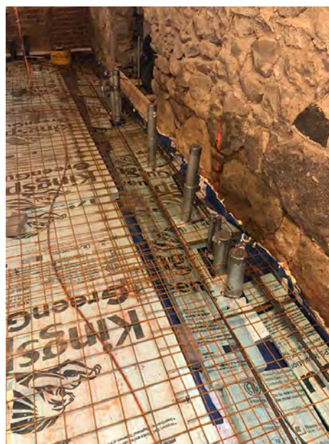
East Wall of Electrical Room with Stubs of Underground Conduits
