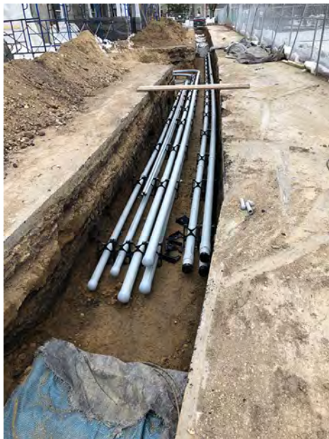
Conduit Installation in Progress
