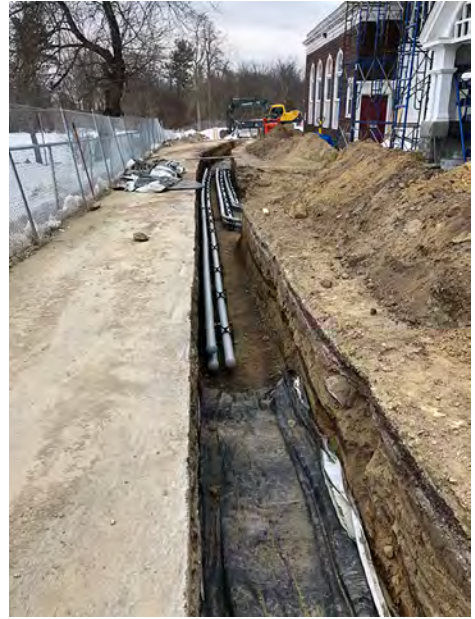
Electrical Service Trench with Conduits in Progress
