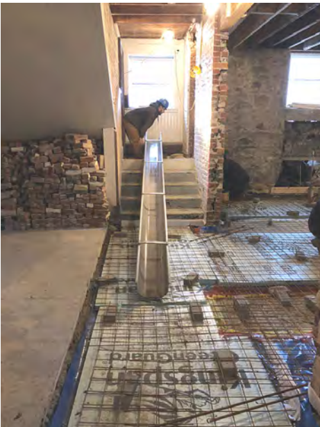
Concrete Chute from East Portico Entrance; Office Area Existing Slab at Left
