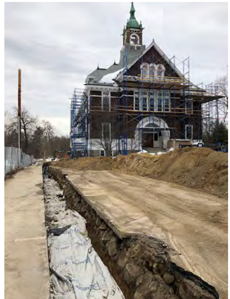
Trenching for Electrical Service at Exit Drive
