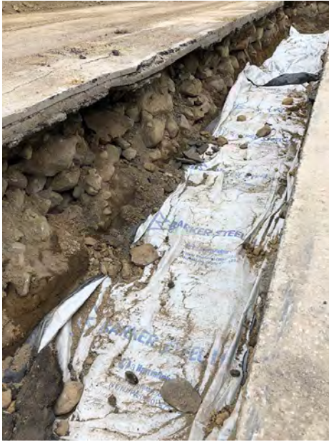
Detail of Excavation Trench at Exit Drive Looking Toward Main Street
