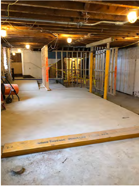
Lower Lobby Slab with Shoring at Elevator Hoistway Beyond
