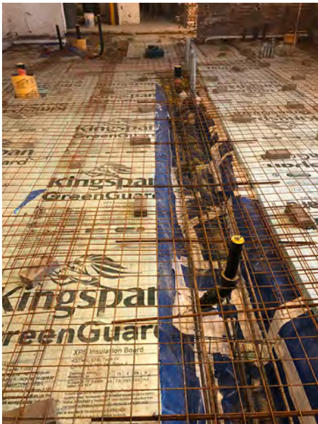
Deeper Trench for Added Bearing Wall to Shorten Original Joist Span at First Floor Above
