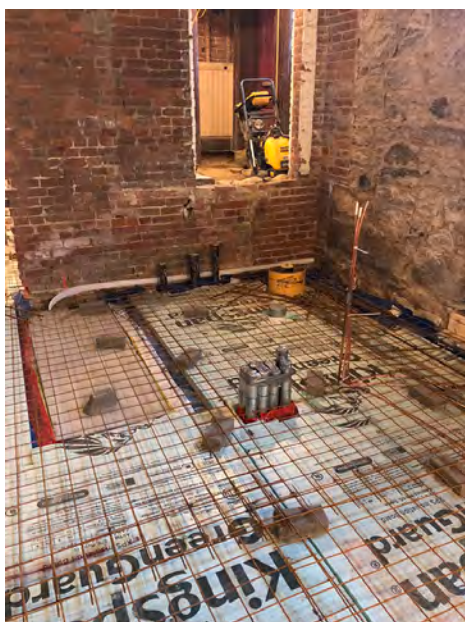
Electrical Room in Foreground Adjacent to Staff Accessible Toilet Room
