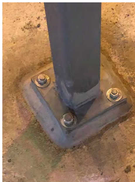
Tube Steel Post and Base at Facility Manager's Office
