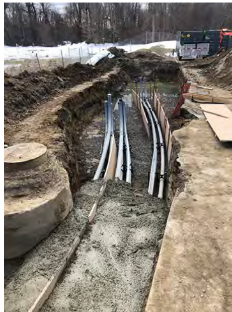
Concrete Coverage in Process at Conduit Trench
