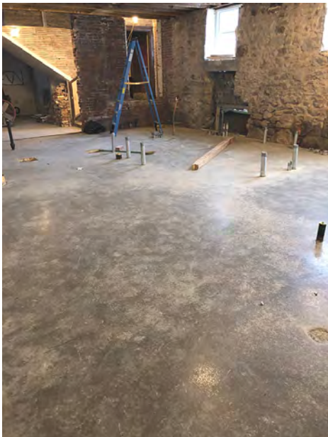
Concrete Slab at East Half of Basement
