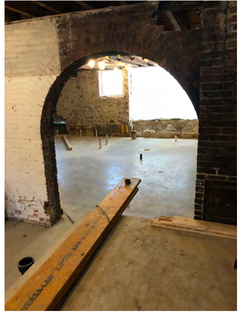
Slab at Lower Lobby Accessible Toilet Room; Archway to Boiler Room Beyond
