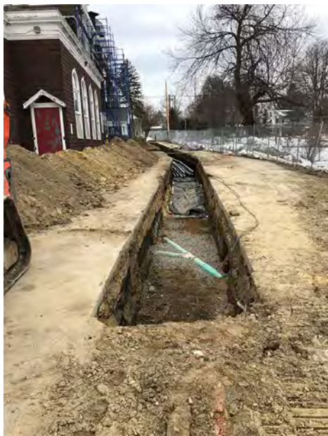
Looking Toward Main Street from South End of Conduit Trench in Vicinity of Transformer
