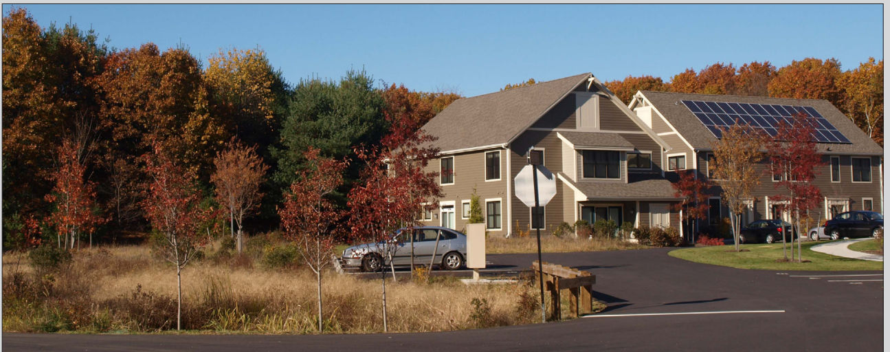
Vegetated drainage basin provides a different buffer
