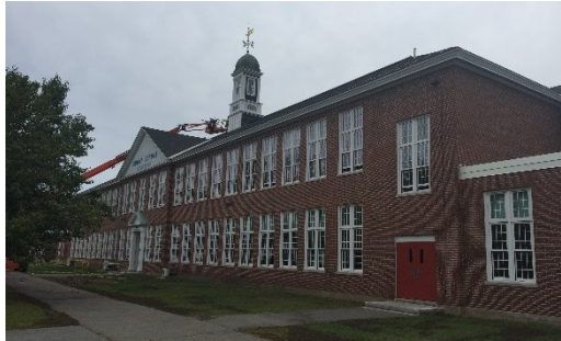
Repairs to the Abbot School cupola were included as part of the project.
