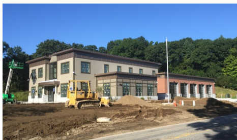
Construction of new Fire Station on Boston Road nearing completion
