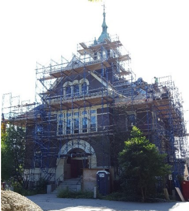
Roudenbush is receiving a new slate roof, exterior paint and extensive repairs to the cupola.
