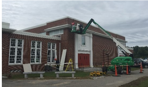
Workers complete installation of new metal fascia at Abbot School gymnasium.
