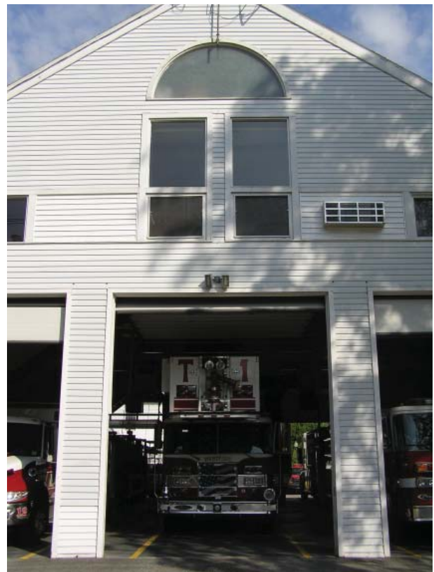
Westford Fire Department Headquarters.
