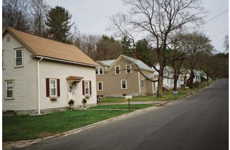
Historic workers' housing, Orchard Street, Forge Village.
